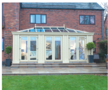
Loggia Glazed Extension
